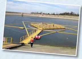
↑ This solar-on-water system also works as a water reservoir cover that helps reduce evaporation and protects the water source.
